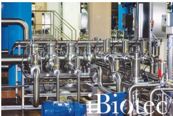
Cleaning of distribution pipeline cloths in the agrifoods industries
